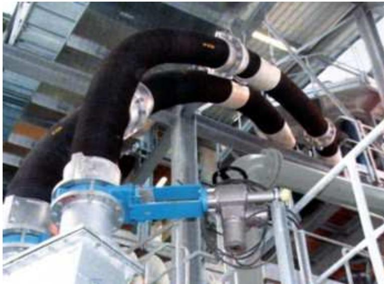
**Hoses, system TT**, for the transport of abrasive materials under wet conditions is conceived being durable and having a long lifetime. The hoses TT are conform highest mechanical solidity and closeness. The system is made up by 3, easy exchangeable, standardized parts: the **TT hose**, the **TT coupling** and the **TT seal**.
