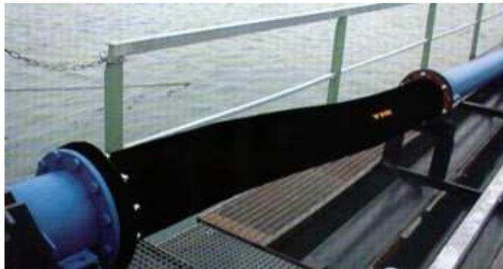
The TT hose system can be installed, as a flexible connection, between tube systems to compensate for shrink or expansion. The rubber hose absorbs all movements, created by temperature or vibrations.
